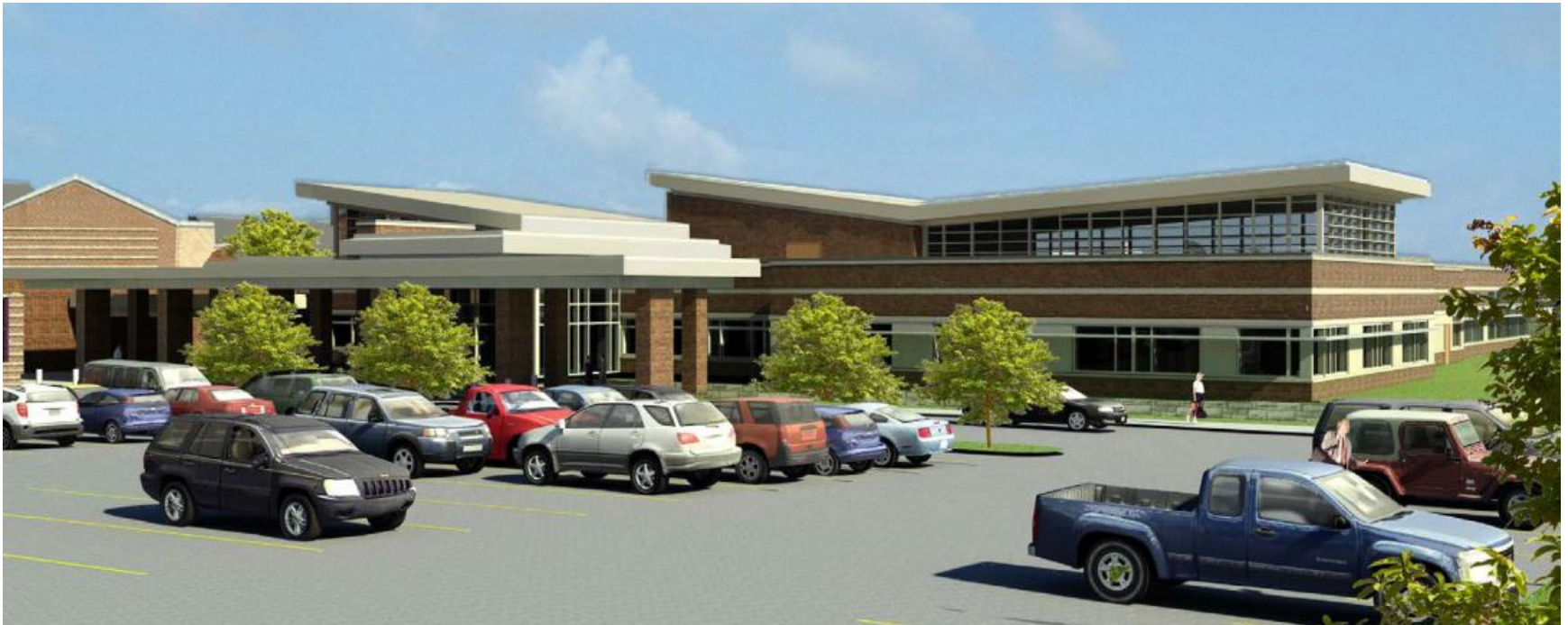
View from North Entry
